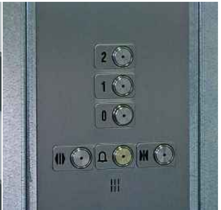
Car control panel of stainless steel, vandal-proof
